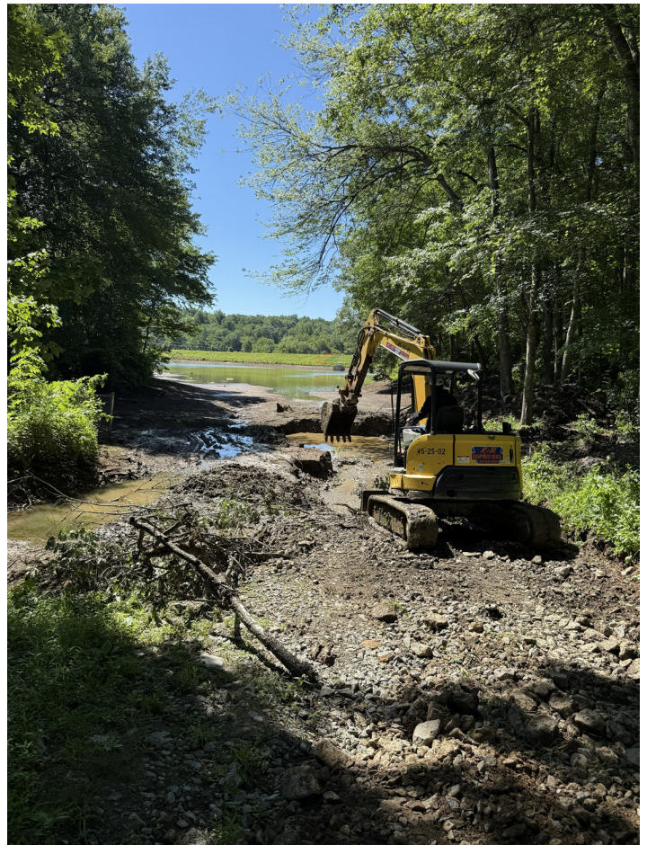
June 13, 2026 - Construction begins on Lake 2 concrete boat ramp.
