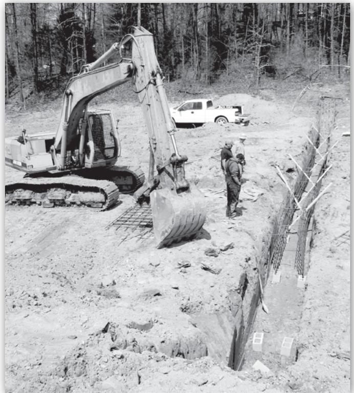
*Construction of a concrete weir for the lake Greene's renovated spillway, engineered to comply to new Virginia State guidelines.*
