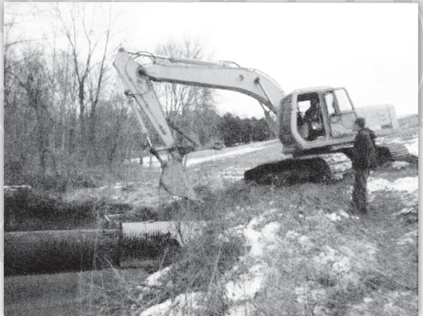
*New HDPE outfall pipe being inserted to line the existing deteriorated outfall pipe.*
