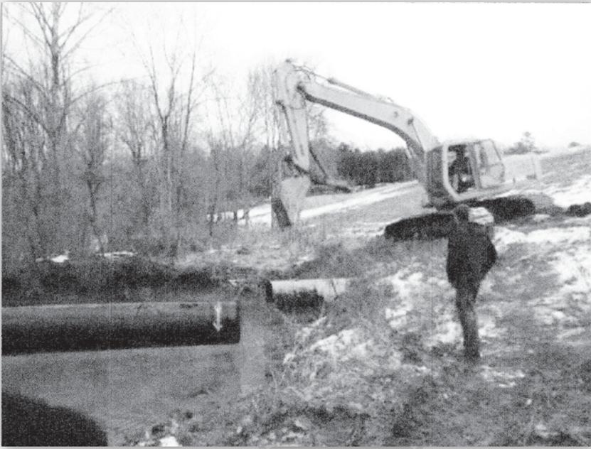
*Bander Smith moving end of the new HDPE outfall pipe into position.*
